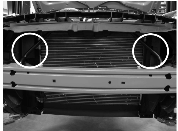
Fig. 5-a: Remove Front Braces
