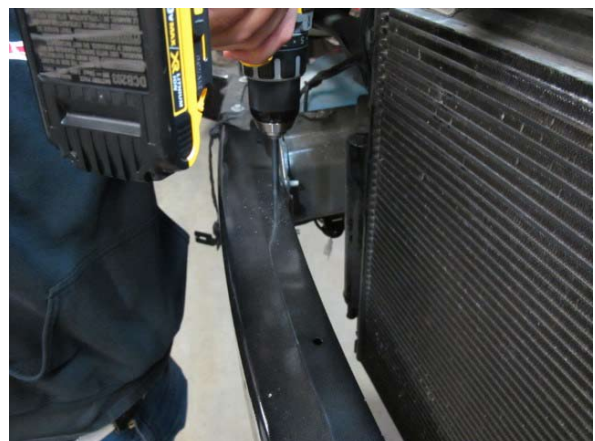
Fig. 7-u: Drill holes in front bumper support
