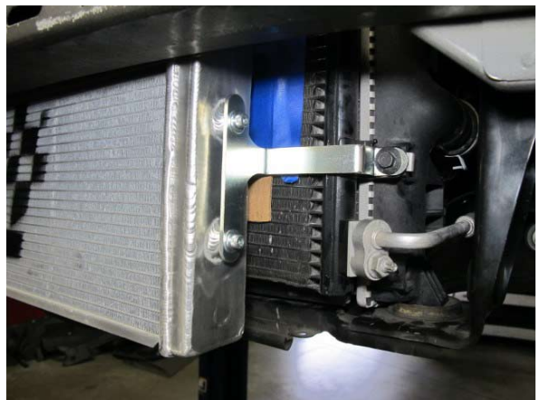
Fig. 7-i: Install driver side of heat exchanger assembly
