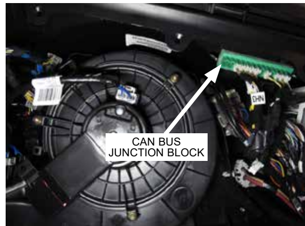
Fig. 14-b: CAN bus junction block
