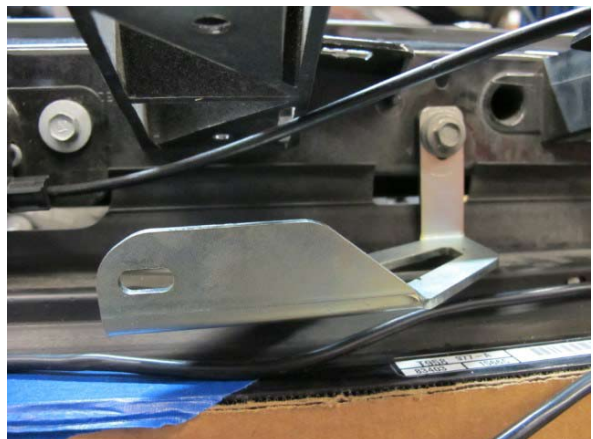
Fig. 7-o: Install upper air/water cooler support bracket
