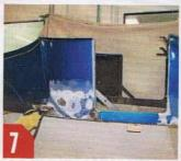
7) When you want to check an area to see what's underneathbe prepared. After blasting off the covering paint there were a number of trouble spots. When blasting it can uncover more work than you bargained for.
