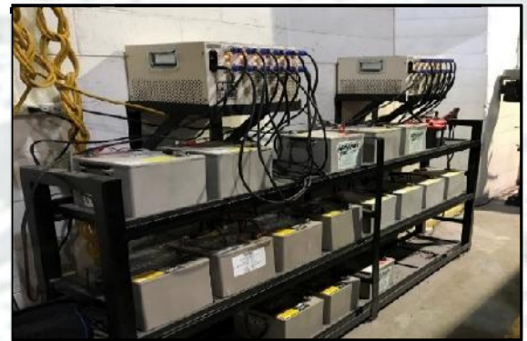
This high-speed unit added brackets, and 2 Pro-PC-12s to upgrade their charging rack capability.
