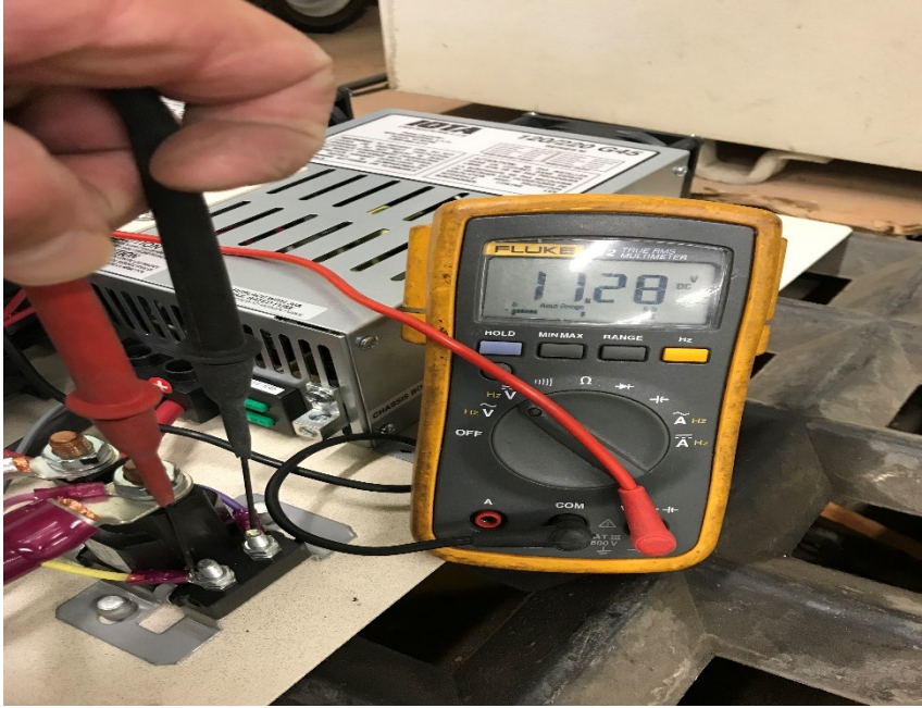
Testing activation VDC on upright solenoid switch.
