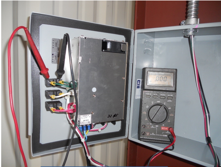
Grid Zone Circuit Breaker test
