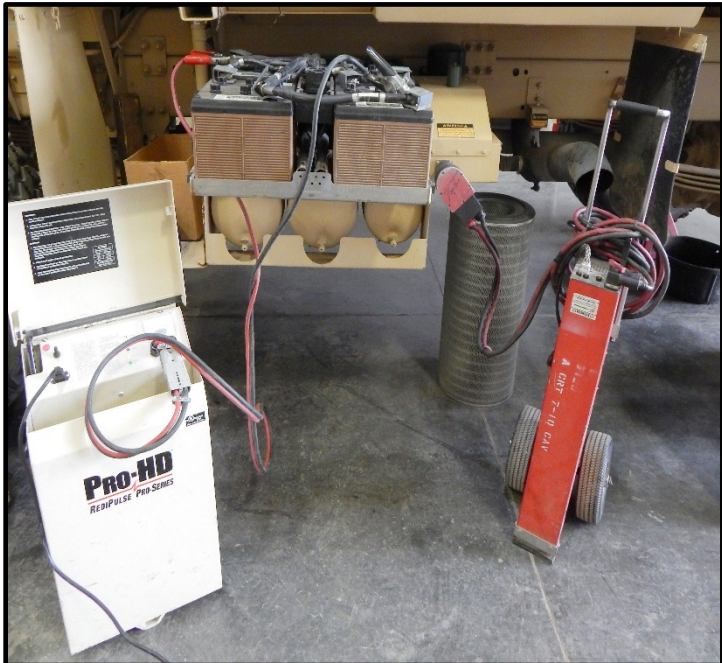
Example: Getting a low VDC or highly sulfated 24VDC system to start charging via a jump start.
