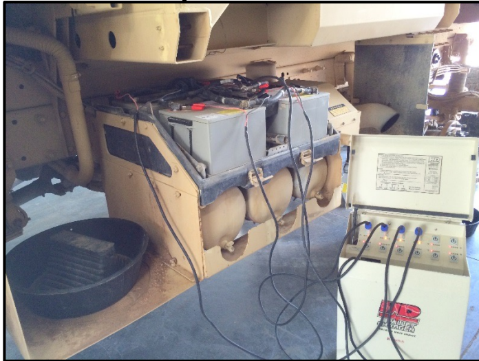
Example: Pallet Charger engaging a 4 battery, series / parallel system.
