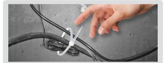
If needed, use plastic cable ties (not included) to secure the circuit box wires to the battery cable or other secure area near the battery. This will keep the wires from being damaged or interfering with any moving engine parts.
