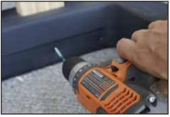
3. Drill 1 screw into each section, through the wood. Do not overtighten.
