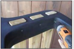
5. Drill 1 screw into each section, through the wood. Do not overtighten.
