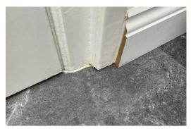
Best practice here would be to undercut the architraves and slide the flooring underneath, allowing the expansion gap to be hidden and maintaining a neat finish – **not** to fill gaps with silicone.
