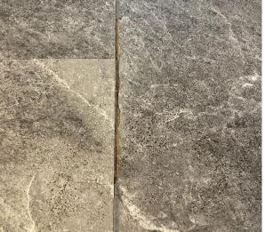
This close-up shows the damage caused to this flooring over time due to unwanted movement underfoot. When first laid in this manner, the flooring will look perfect, but the movement breaks down the joints of the click system which will eventually begin to separate like this. Remember that **SPC flooring has a rigid core and should not move underfoot**.
