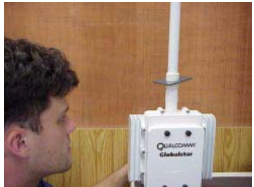
Figure 6. Locating possible obstructions
