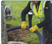
Perforated pipe is fitted as a loop, which is installed 200-300mm below the surface at the outer circumference of the rootball on all trees 150 litres or above.
