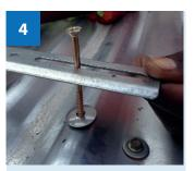
Fit single universal fixing bracket with roof sealing washer and screw.
