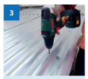
Locate batton where panel will be fixed on. Drill 6mm hole on high end of roof.
