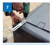
Fit double universal fixing bracket to the bottom of the geyser using supplied 6mm self tappers.
