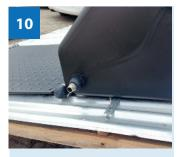
Put geyser on place over panel and fix brackets to the brandering.
