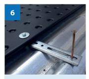
Place collector on bracket and attach using nut and washer. ON LEFT AND RIGHT SIDE OF PANEL USING CENTRE HOLE.
