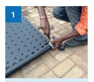
Attach solar connector and stop end using supplied hose clamps.
