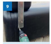
Fit cistern tank onto geyser using supplied 4mm self tappers.
