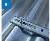
Place cupsquare under universal fixing bracket with threaded section pointing upward.
