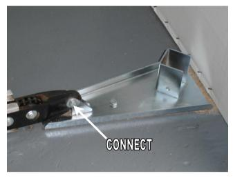
Mount the head bracket and wall bracket to each other and then to the garage door motor with the bolts and nuts provided. See picture below.
