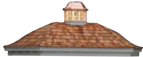
Cedar Shake Roof
