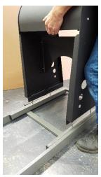
Step 6: lower barrel assembly onto clamp bolts and slide in either direction until side panels are stopped against the bolts.
