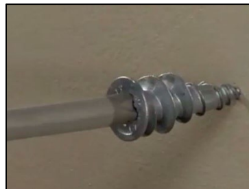
Figure 3. Installing drywall anchors
