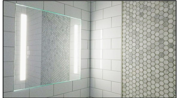
Figure 4. Grout around the mirror to seal and finish.
