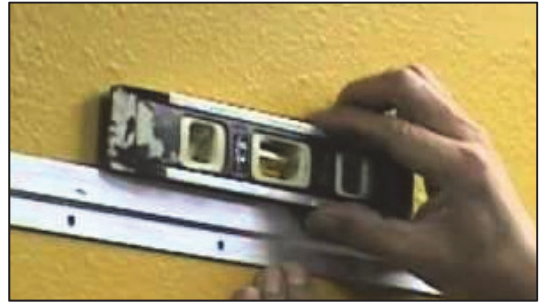
Figure 3. Level and Mount Z-Bracket Wall Plate.
