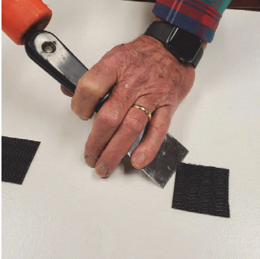
Figure 9. Removing the Dual Lock patches from the wall.
