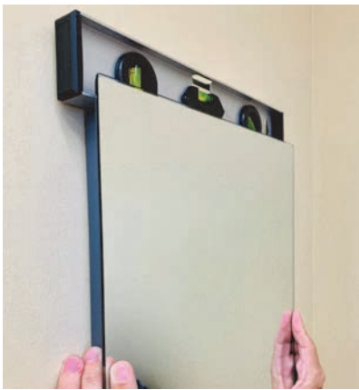
Figure 5. Position, level and snap in place.
