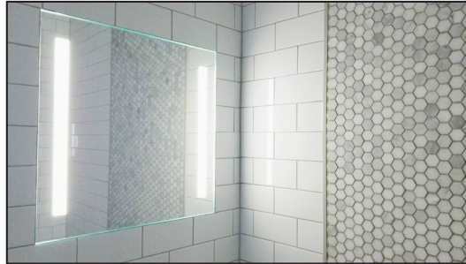
Figure 3. Grout around the mirror to seal and finish.
