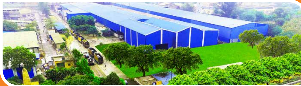
Sikanderabad, Uttar Pradesh (Unit-I)
