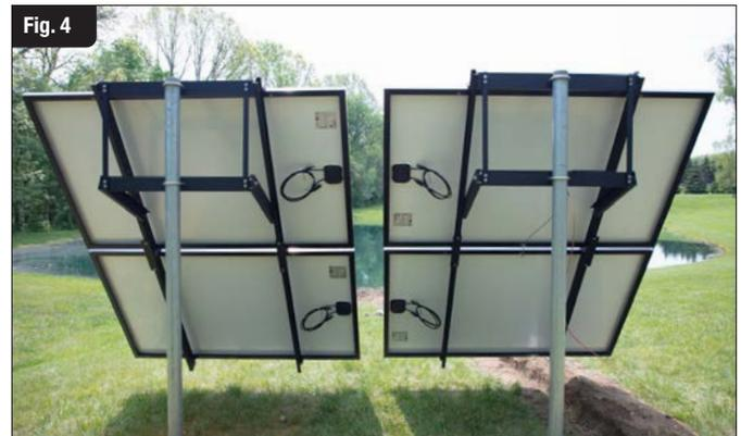
5) Next, loosen the double-sided clamp from the rail on each side. Then position the clamps so that they seat against the top frame of the solar panel. Secure clamps to the rail but leave the top hex bolt loose to allow for positioning of the next solar panel (**Fig. 5**).
