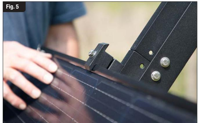
6) Position the second solar panel atop the double-sided clamps, making sure that the wiring junction box faces the same direction as the lower panel and hand tighten. Then slide the top two single-sided clamps down until they seat against the top frame of the upper solar panel. Secure the clamp to the rail with a 7/16" wrench, but leave the top hex bolts only hand tight (**Fig. 6**).
