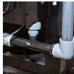
Mazzei® venturi air injection system sustains beneficial aerobic microbes while preventing bacteria from turning odorous and anaerobic
