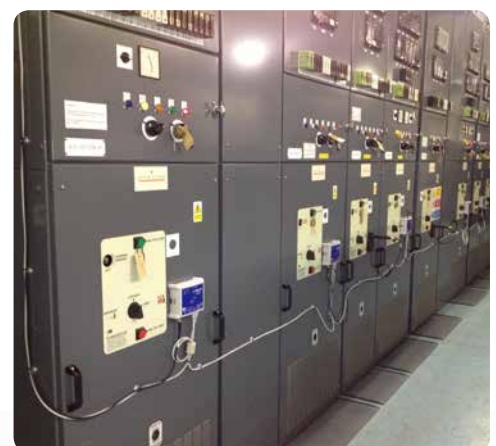
Installation at Dow Corning Site
