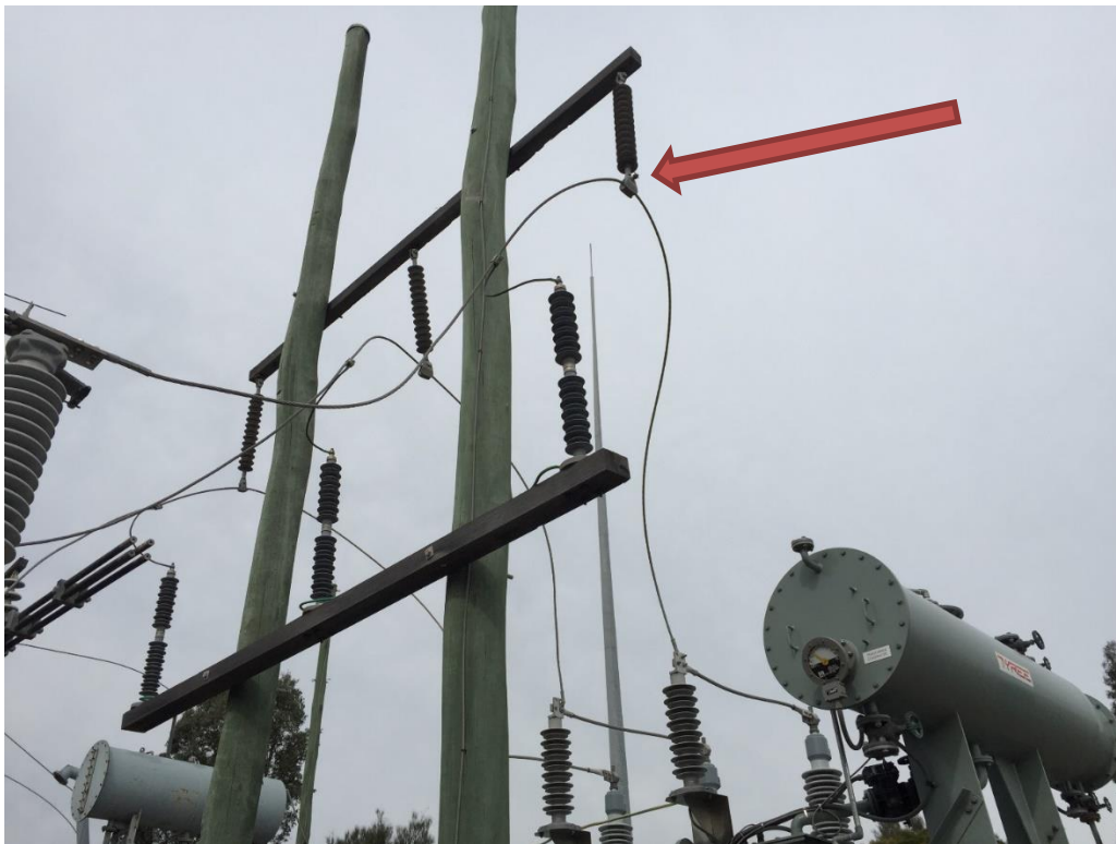
Figure 7 North phase 66kV dropper at TX021
