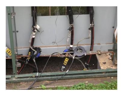
Figure 9. Real-world example of RFCT connection in the United States
