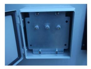
Figure 10. External Test Box wired to permanently mounted RFCTs
