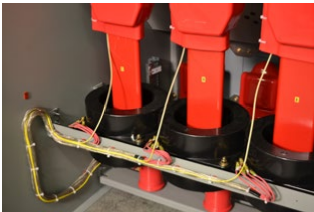
Figure 18 Completed Fiber Installation
