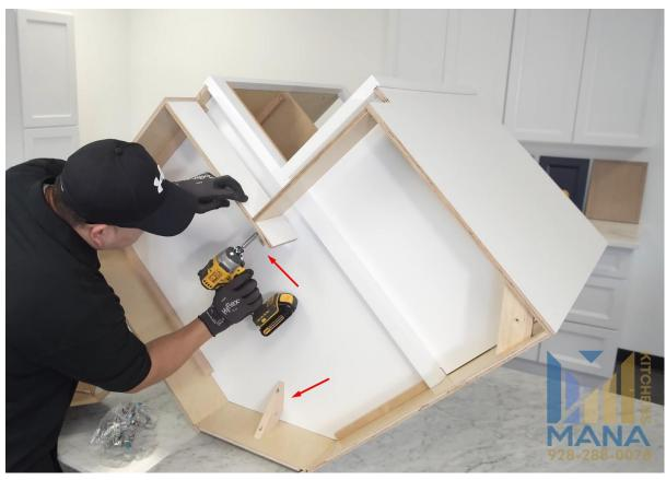
11. Turn the cabinet back on its "feets" and tighten the face frame with remaining holes and screws.
