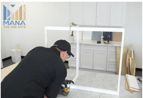
2. Install cam lock metal clips on both parts of the frame as shown in pictures below.
