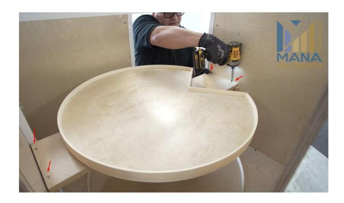
7. Slide in the small back piece and attach it with screws Pictures below
