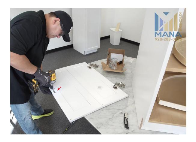
2. Attach the doors with hinges to the cabinet as shown in the pictures below.
