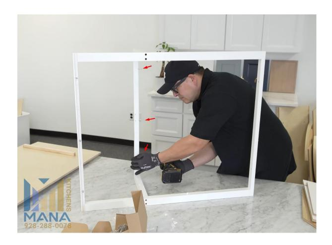
3. Attach metal brackets to both side panels. (Brackets should be added to side opposite from the side where predrilled holes for cam locks are) Please see the pictures below.
