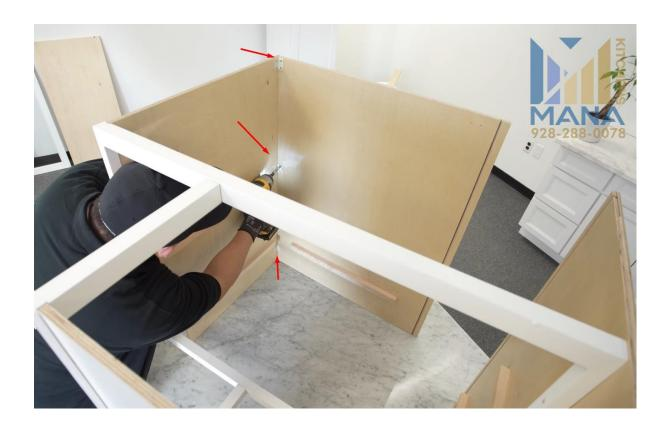
6. Insert bottom panel and shelf with trays and attach them with screws as shown in the pictures below.
