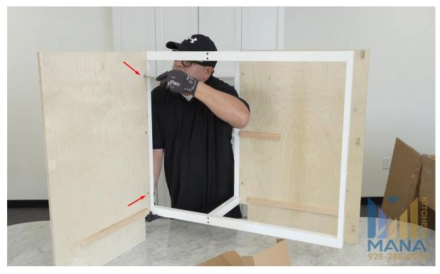
5. Attach back panels to the side panels with L brackets. See pictures below
