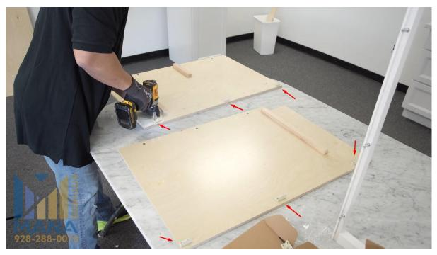
4. Attach side panels to the frame as shown in pictures below and insert cam locks to predrilled holes. (When panels are connected tightly with the face frame lock the cam locks by turning them clockwise)
