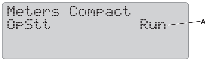
Figure 18: Overview of the menu Meters Compact for the status of the Sunny Island inverter
