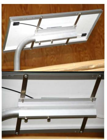
2. Secure pole mounts to building side, attach panel to mounting pole, align to true north, and tighten locking bolts:
