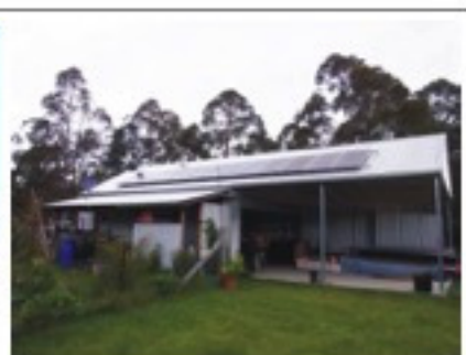
Solar panels flat mounted
