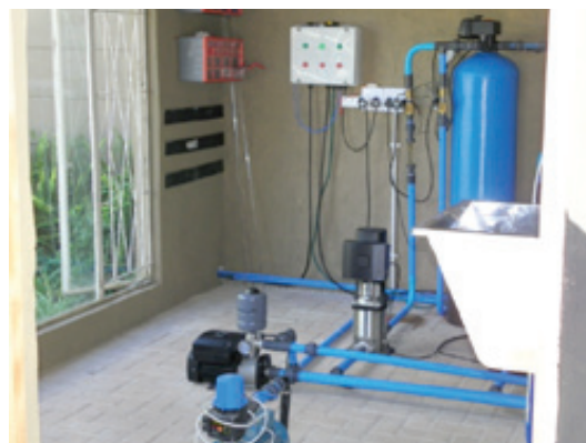
Solar surface CR pumps with the MGFlex motor, from an installation in South Africa
