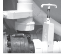
Slice Valve and Pump Union
