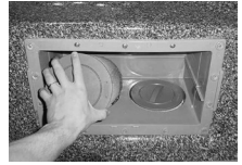
Turn Filter Counter-clockwise to Remove
