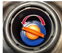
Turn Filters Counter-clockwise to Remove
