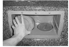
Turn Filter Counter-clockwise to Remove
