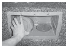
Install Eco Pur filter on left side.
