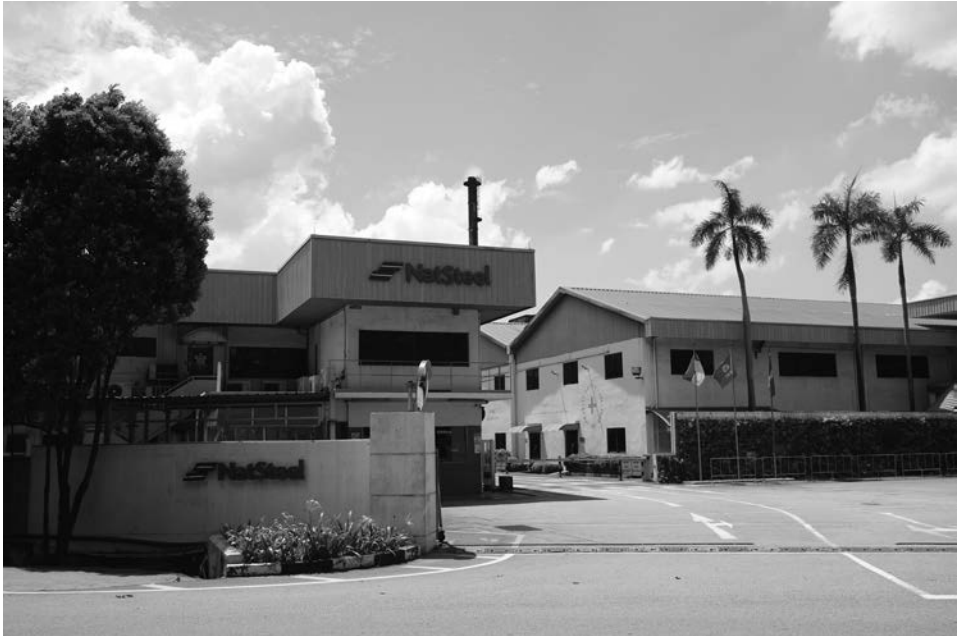
National Iron and Steel Mills (now NatSteel) at Tanjong Kling Road in Jurong Industrial Estate, 2018. Photograph by Juria Toramae.
