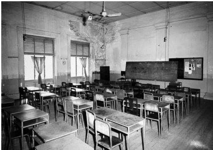
One of the classrooms at Bras Basah Road RI
