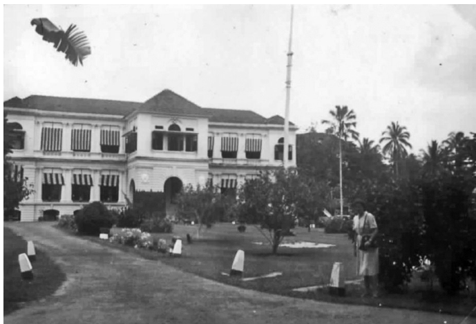
The Sultan's palace, Pekan, 1954 (photo credit: Jean Marshall)
