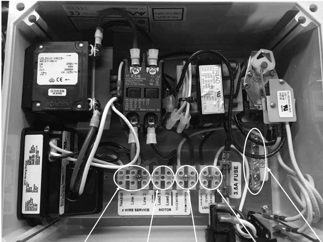
Figure 24 Control Box Wiring Connections
