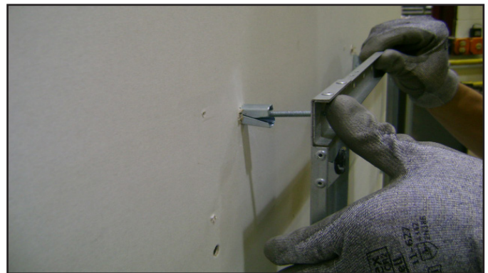
Figure 4.11 Installing Anchors in Hollow Wall
