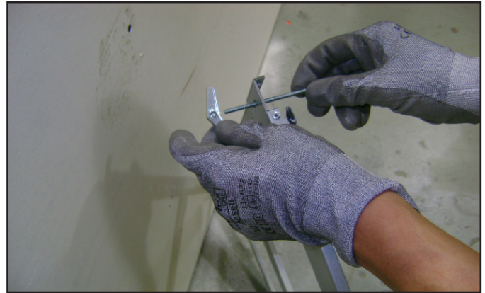
Figure 4.10 Toggle Bolt Installation through Mounting Bracket
