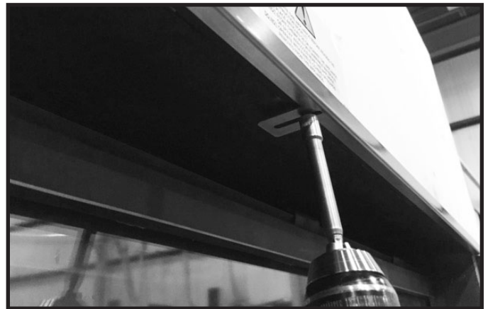
Figure 10.5 Install Trim Ring
