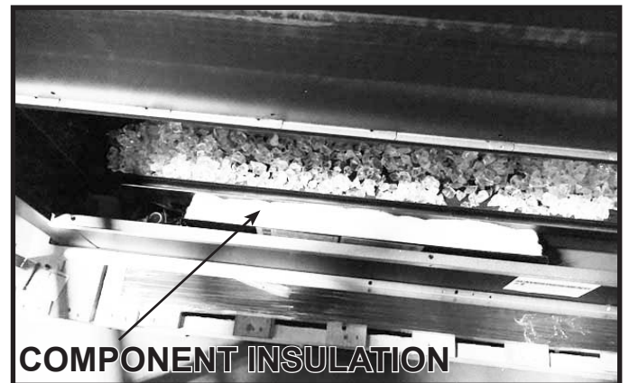
Figure 11.3 Component Insulation Location
