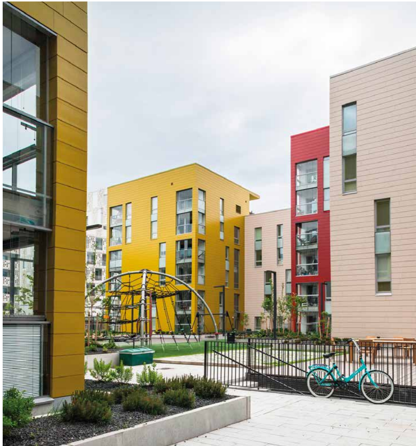
tempio® [projects] Saukonkanava, Helsinki, Finland.
