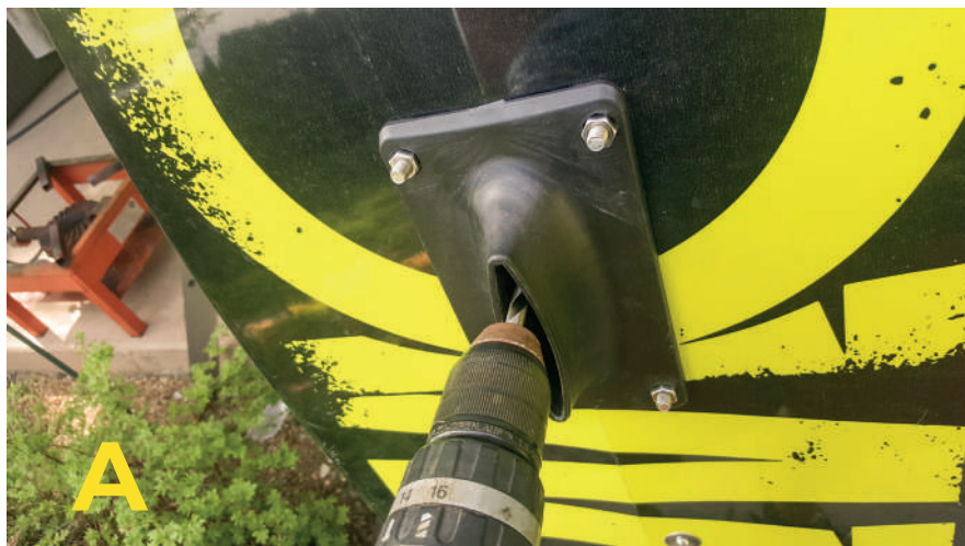
DRILL 8mm MAST SCREW HOLE USING BASE MAST AS A TEMPLATE
