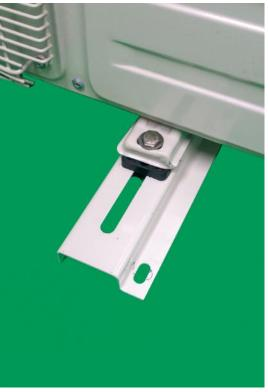
The system is now mounted to the bracket. Feet holes are available for mounting to a pad/slab.
