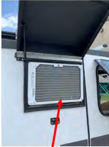
AC shroud shown open AC must be unlocked and pushed out from interior of habitat
