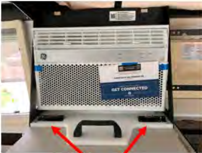
AC driving locks Both locks must be engaged for driving
