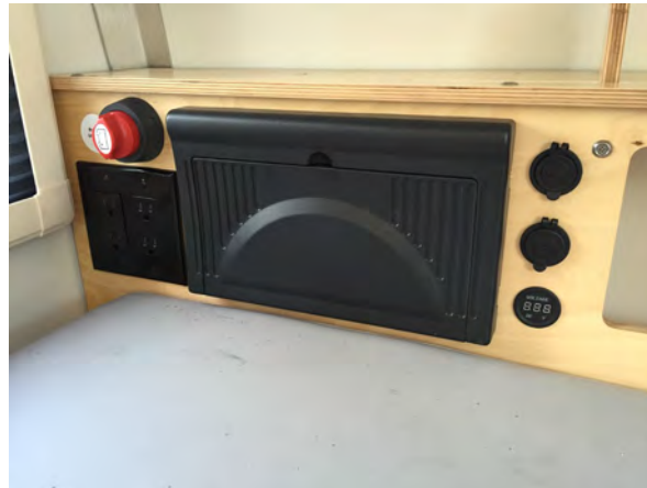
Battery Cut Off Switch / 120V Outlets/ WFCO power center / 12V outlet / USB Outlet / Voltmeter
